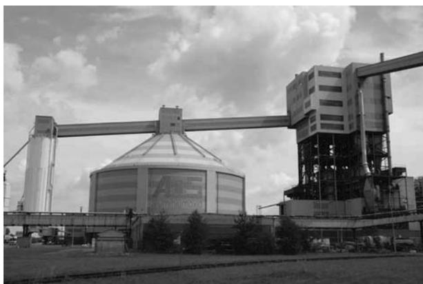
Figure 1. Calciners and alumina storage silo at AOS.
