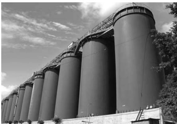
Fig.5. Precipitators of 4500 m3 with advanced mechanical agitators
