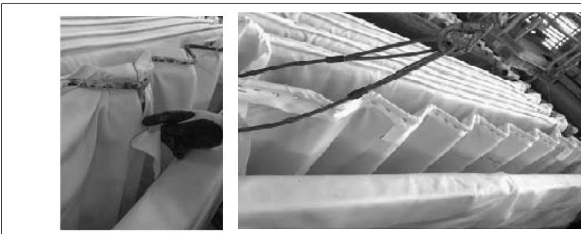
Photographs of the re-clothing procedure and bag/frame ready for service
