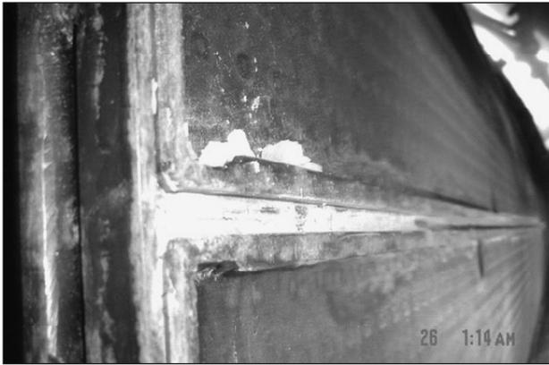
Figure 6. Scale formation in metal profile corners
