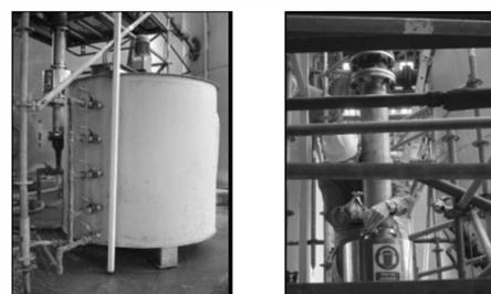
Figure 5: Left: 2m<sup>3</sup> temperature controlled stirred tank; Right: Installation of the C<sup>3</sup> 5L ultrasonic flow-cell
