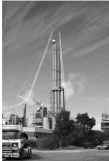
Figure 3 — Calciner Multiflue Stacks
