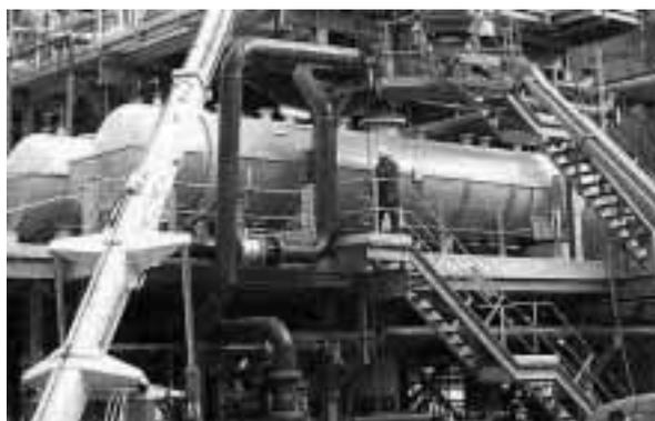
Figure 6 — Digestion Vapour Condensers
